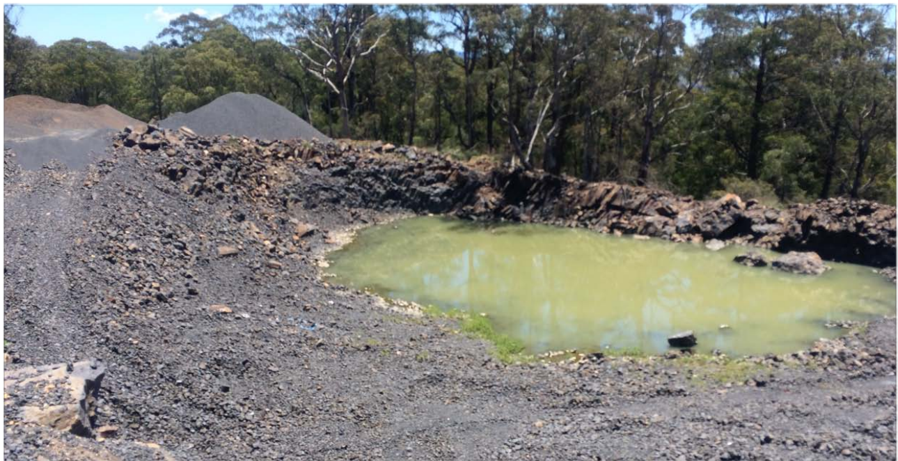
PHOTO 4: Existing quarry sediment dam- approx. depth 4m. No extraction beyond steel posts
