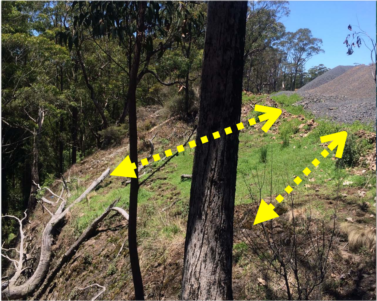
PHOTO 8: steel posts have been placed within 10m-15m of the steep rocky scarp (indicated by yellow broken lines/arrows), on the northern boundary of the quarry, in order to protect areas downslope from the impacts of quarrying- refer Section 2.1 of this Annual Review.
